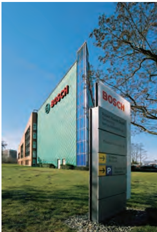
Bosch Engineering Sales Office Braunschweig
